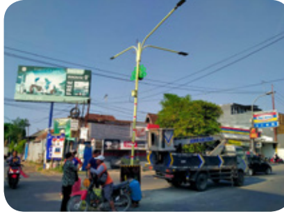
Pemasangan lampu jalanan Installation of street lights
